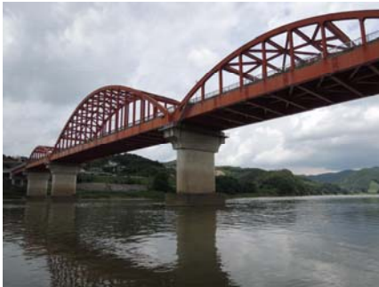
Fig. 7. Bulti Bridge, the Republic of Korea.
