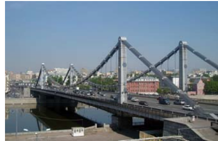
Fig. 5. Krimskiy Bridge in Moscow.
